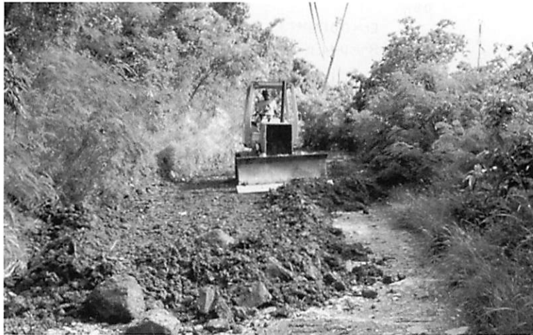
Figure 7. Example of a grading operation along road segment FB-Coco on 11 December 1998.
