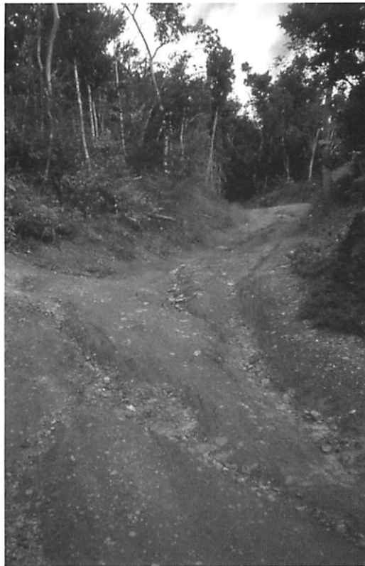
Figure 2. A typical steep road segment near Bordeaux Mountain with a deeply rilled travelway.
